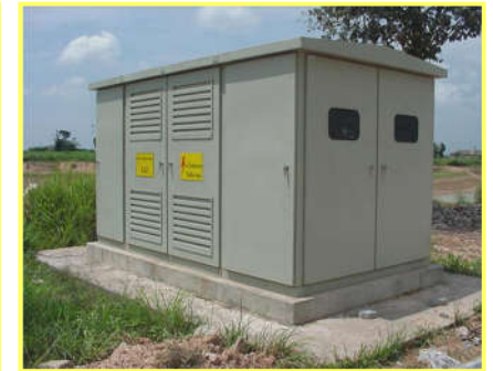
Unit Substation
