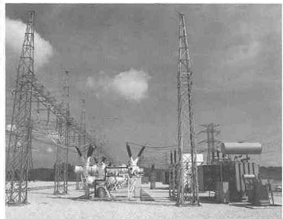
รูป OUTDOOR SUBSTATION
