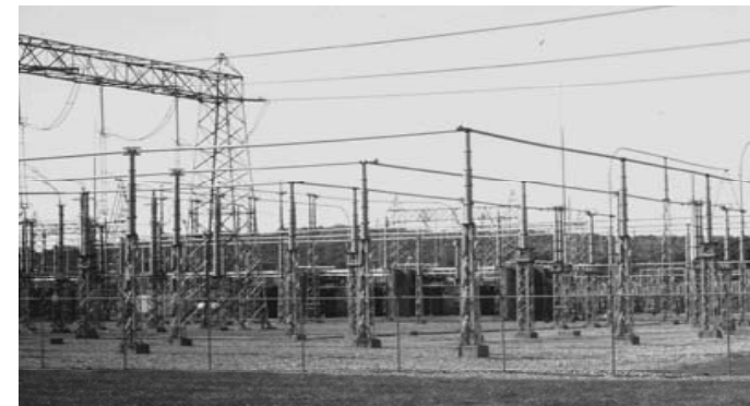
Photo 1. A very large high voltage substation.
