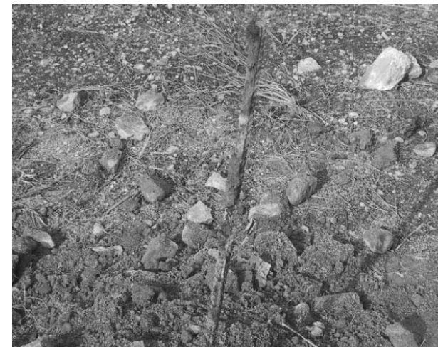
Fig.2. Corrosion of the Grounding Grid
