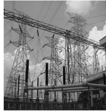
Substation Building and Transmission Lines Serving Substation
